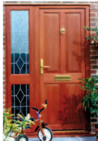
Front door with raised and fielded panels and a full height leaded sidelight. The sidelight midrail aligns with this door but the head and kick rails do not
